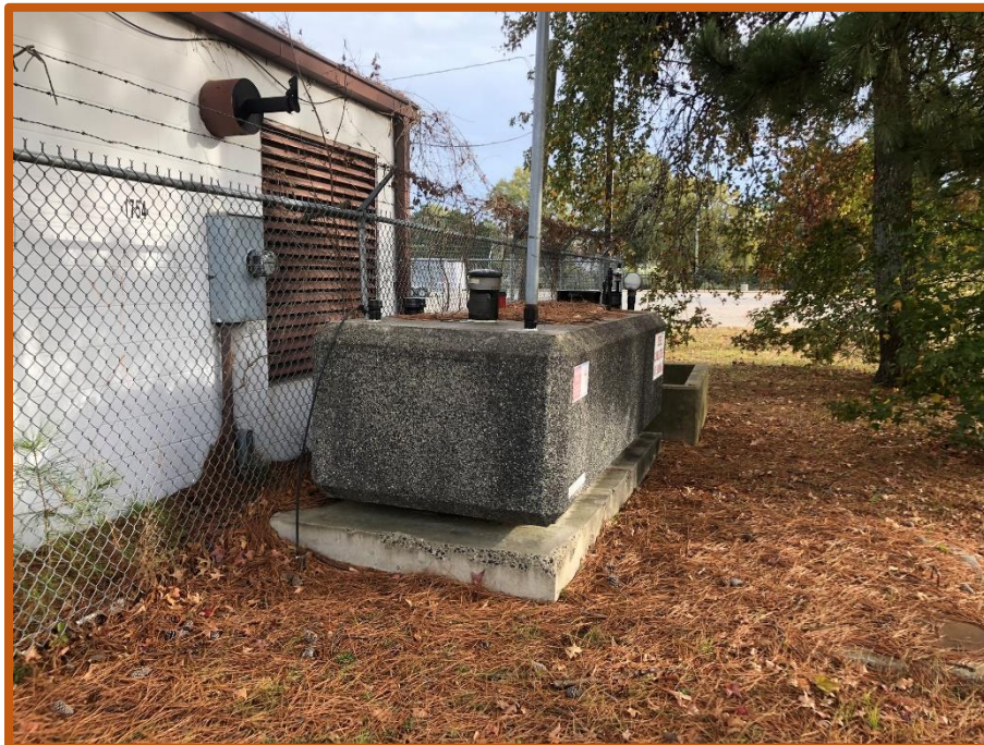
Photograph 10. Typical Emergency Generator with Separate Tank
