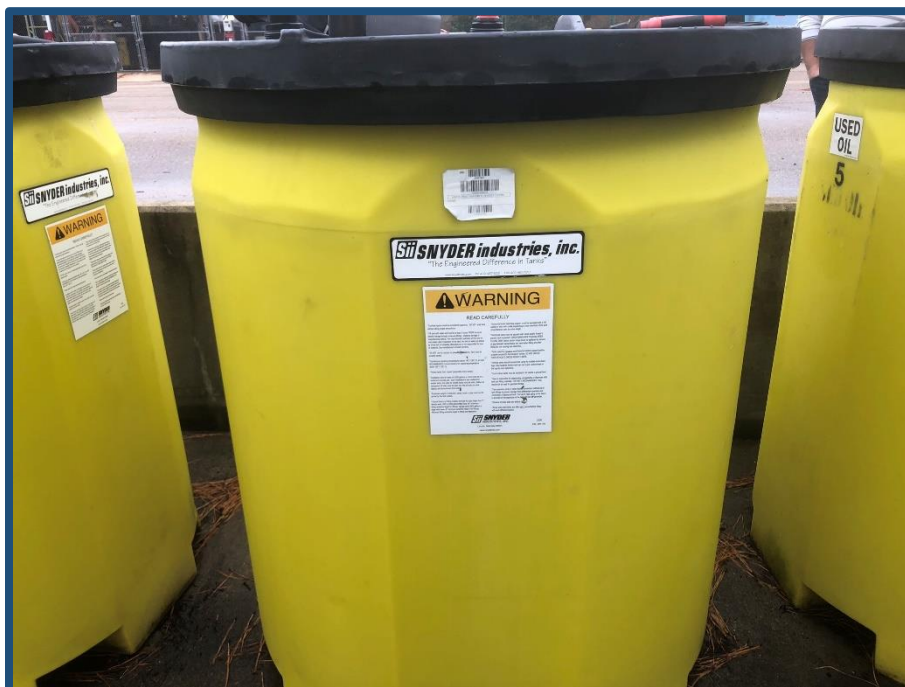
Photograph 5. James River Reserve Area Typical 275-Gallon Used Oil AST (2606-3, 2606-4, 2606-5, and 2606-6)
