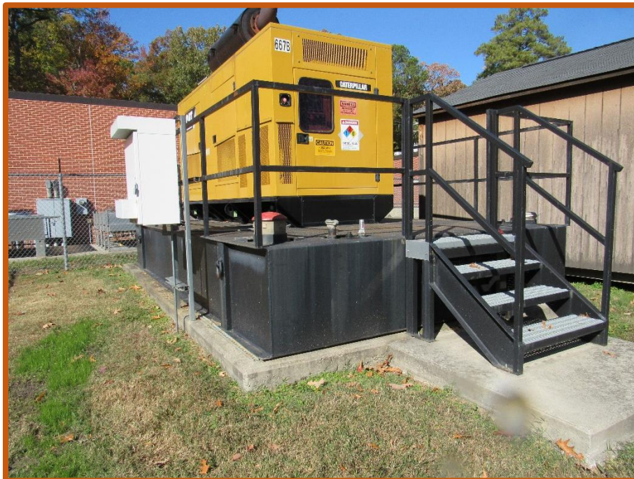
Photograph 9. Typical Large Emergency Generator with Integral Sub-Base Tank
