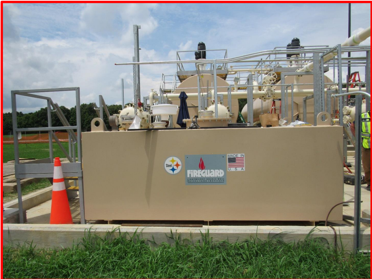
Photograph 2. New Felker Army Airfield Jet Fuel F-24 ASTs
