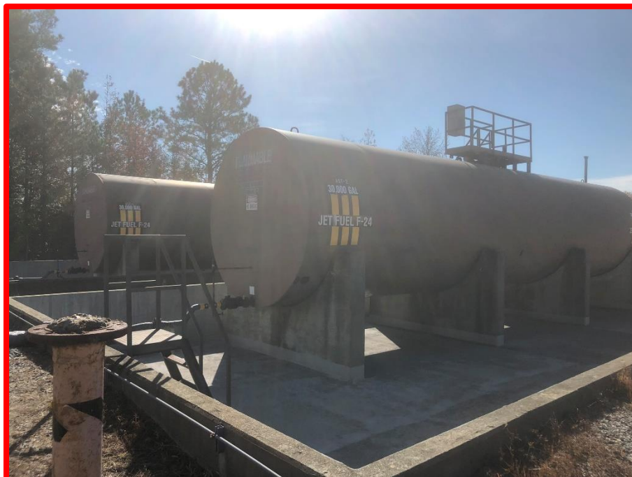
Photograph 1. Felker Army Airfield Fuel Terminal 30,000-Gallon Jet Fuel F-24 ASTs
