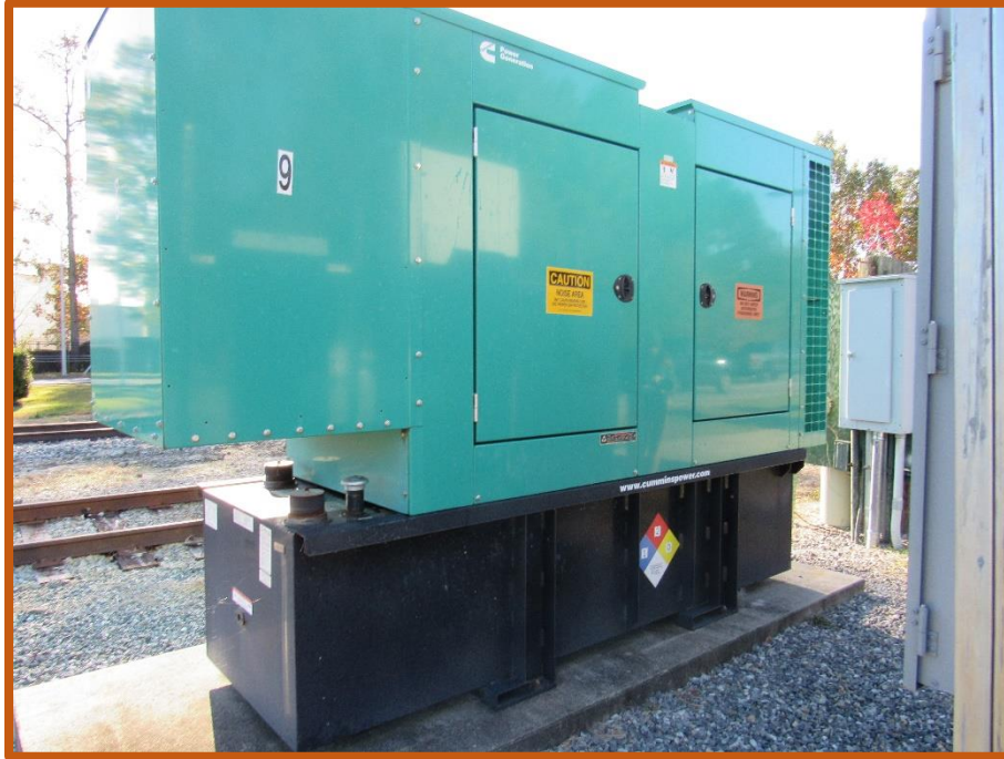
Photograph 8. Typical Small Emergency Generator with Integral Sub-Base Tank
